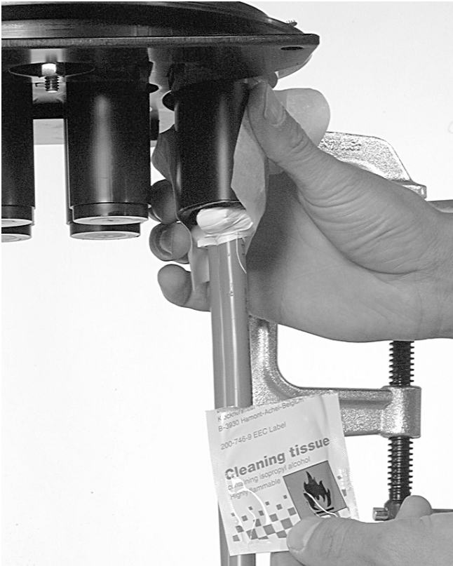
5.1.2 Clean and abrade the cable.
