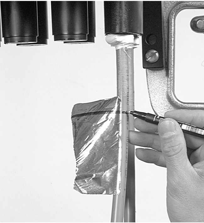
5.1.4 Match the blue line of the aluminium protection foil with the marks on the cables. Wrap aluminium cable protection foil around the cable (the aluminium foil should not be more than 30 mm inside the sleeve).
